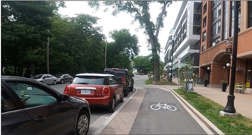
Figure 2: The Halifax South Park Street bike lane includes a short, raised section with curb protection, like those found in Seville. The design still puts cyclists in danger through proximity with the door zone and risk of obstruction from people exiting from parked cars (image credit: the authors).
