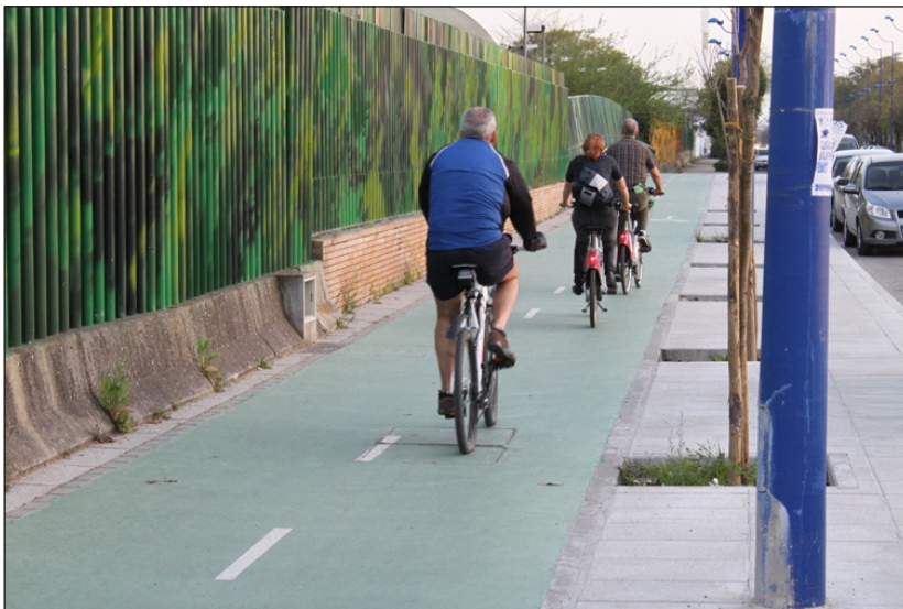
Figure 1: Seville’s visible, connected, and consistent bike lanes include a distinctive green surface to differentiate them from sidewalks and roads (Image credit: Bike Texas via Flickr).
