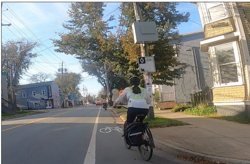
Figure 3: Key parts of Halifax's bicycle network still rely heavily on painted bike lanes that offer no protection to cyclists from parked or moving vehicles, such as this one on Windsor Street (image credit: the authors).
