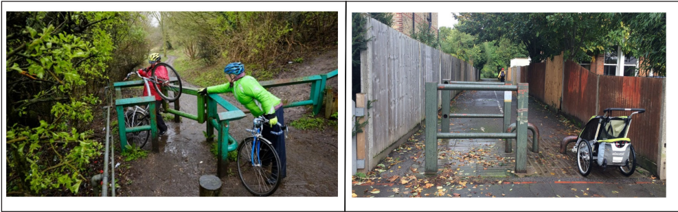
Figure 1: Cyclists struggle to pass through a barrier on the NCN (left); and pushchair unable to access footpath due to barrier obstructions (right). The barrier to the footpath (left of right image) is too tight to fit past, whilst the barrier to the cycleway (right of right image) is designed only for two-wheel cycles. This barrier type, known as a kissing gate, requires a user to manoeuvre around a heavy swinging gate which is not designed to accommodate cycles, wheelchairs or other mobility devices. Photos: Sustrans, 2020 and 2021b.
